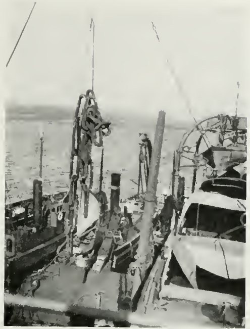
LIFTING CHAIN CABLES.
